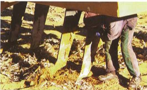
Ripping is done with a twin ripper—the second one rips deeper than the first.
